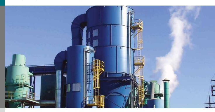
As the cost of energy continues to increase, plant managers are continually looking for ways to reduce power consumption. Part of the Schenck Process filter portfolio is the unique MCF PowerSaver®, a dust collector that can save up to 50% of operational costs by using medium pressure air at only 7 psi for the cleaning cycle. The air is provided by its own blower, therefore no plant compressed air is used, potentially freeing up the expense to produce air for other applications.
